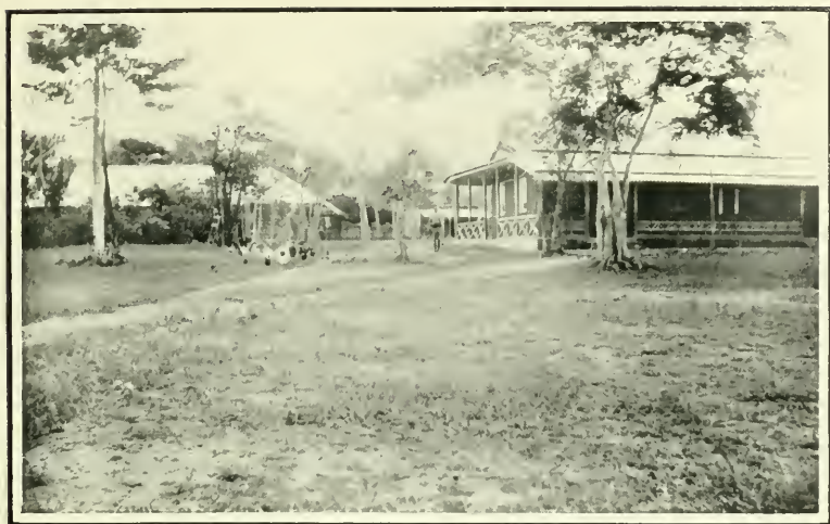
BARRACKS OF THE W.A.F.F. AT DARU
